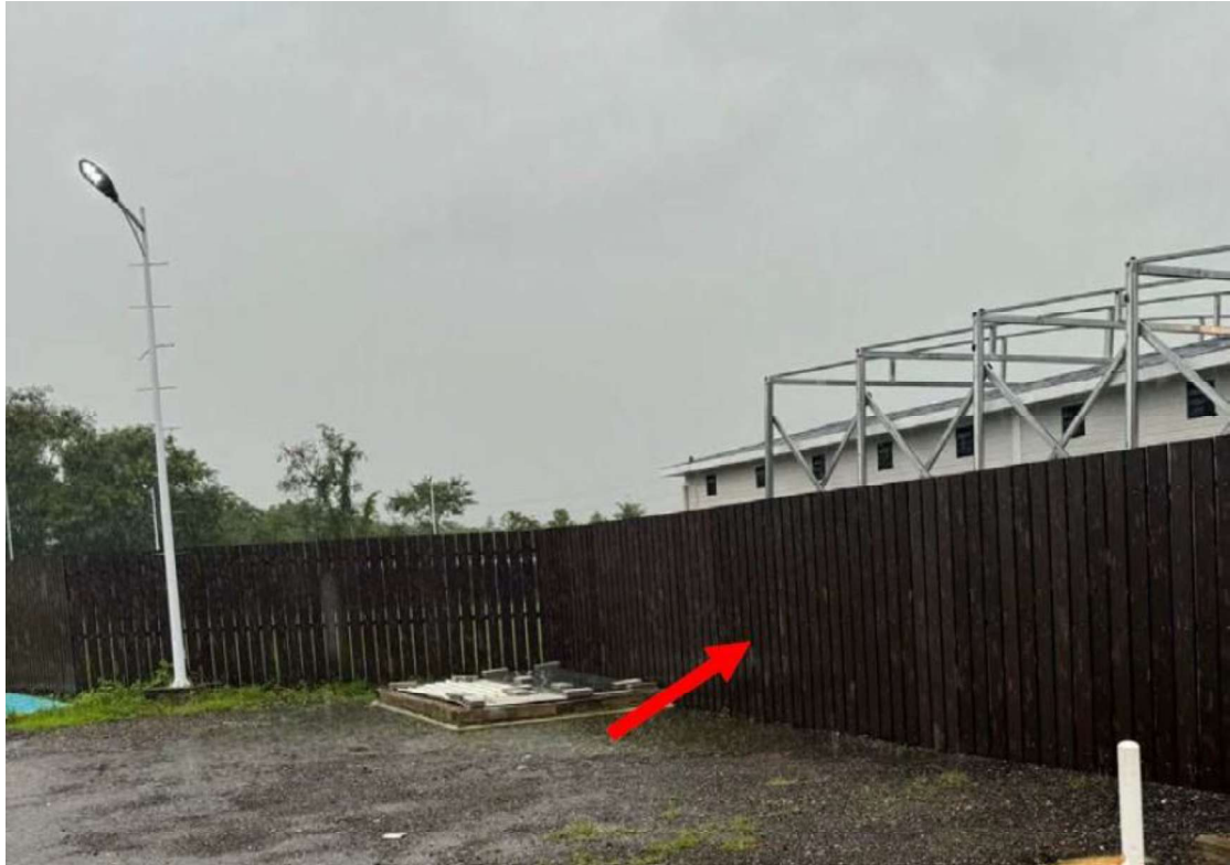
P1 - Fence Wall of Lots No.21, 22 & 28 in DD109
